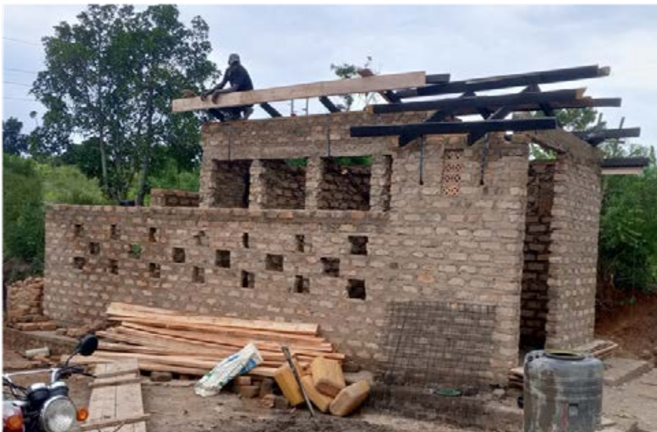
One of the lined pit latrines under construction at the Youth Skilling Centre site
